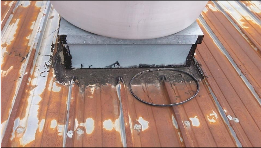
Roofing cement applied around exhaust vent.
